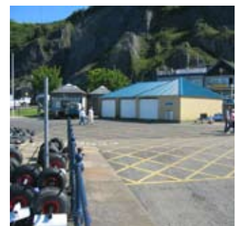
Existing facilities, Knab Rock
